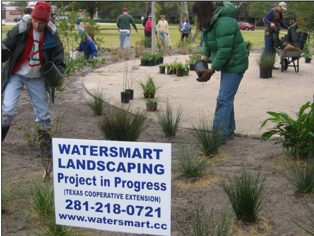
December 2005—Volunteers installing rain garden
