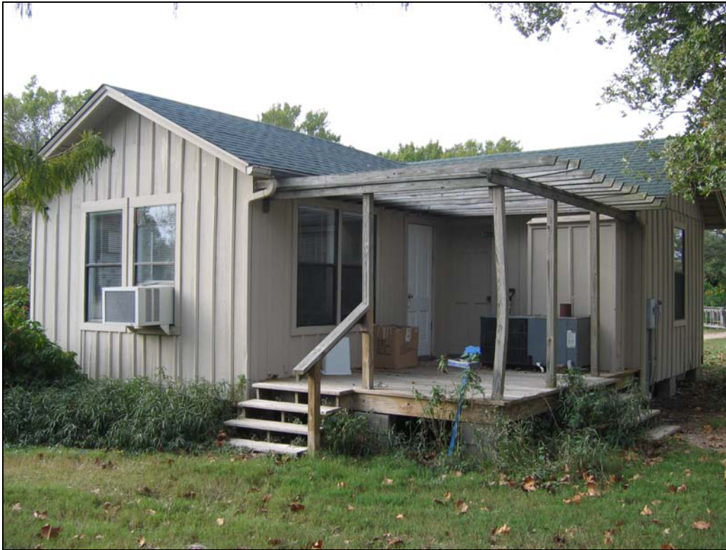
Heiman House—housing education offices--(before photo)
