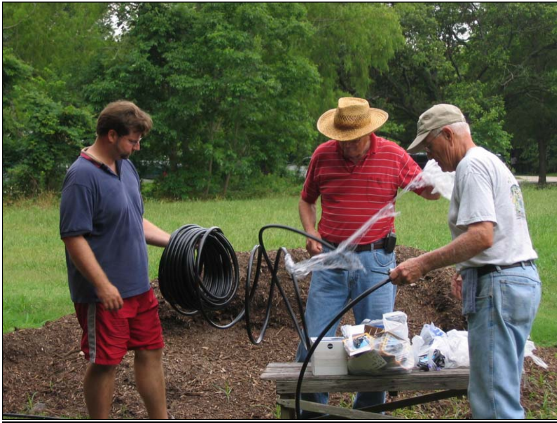
Volunteers installing low volume irrigation
