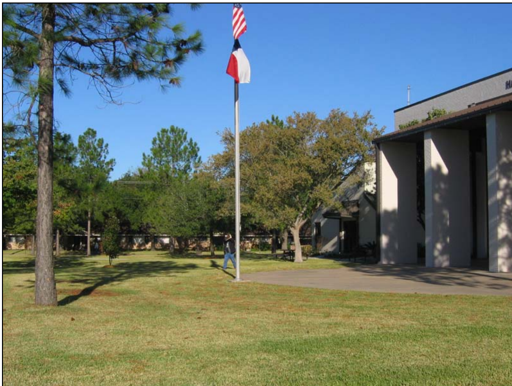
Bay Area Courthouse Annex, Clear Lake Before construction of the rain garden
