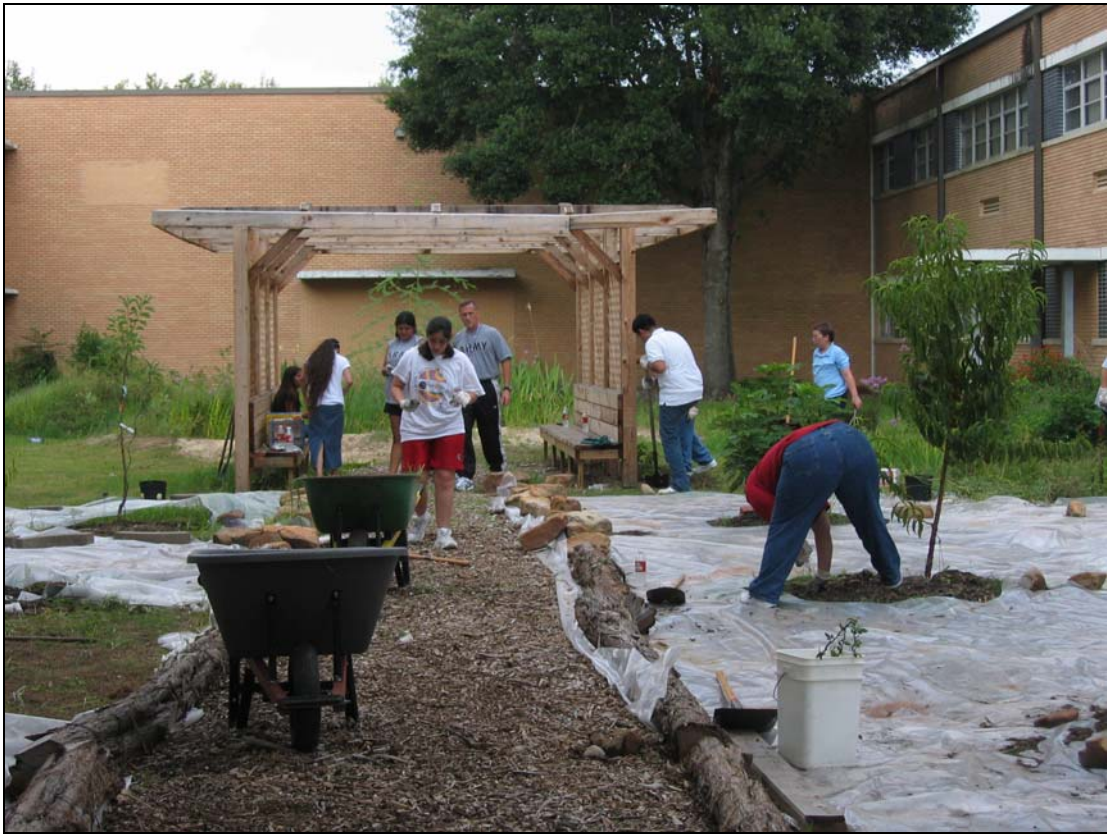
Preparing the site for wildflower seed sowing after “solarization” of the lawn area (Clear plastic sheeting is shown covering lawn area)
