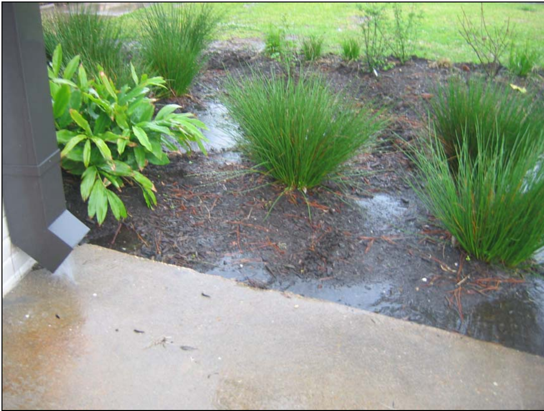
Rain garden in action--collecting runoff from Courthouse roof
